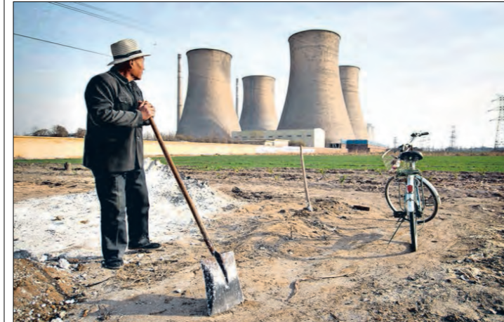
A worker looks at a power plant in Xingtai, Hebei province, where government officials' promotion will no longer be linked to GDP
